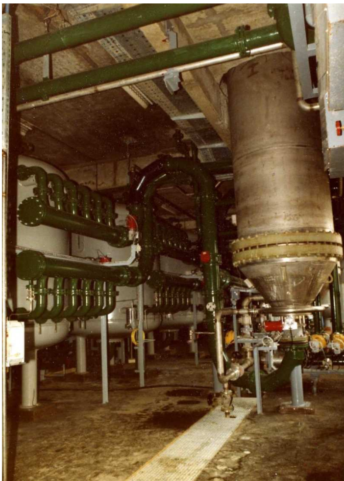
CATION RESIN EXTERNAL REGENERATION COLUMN
