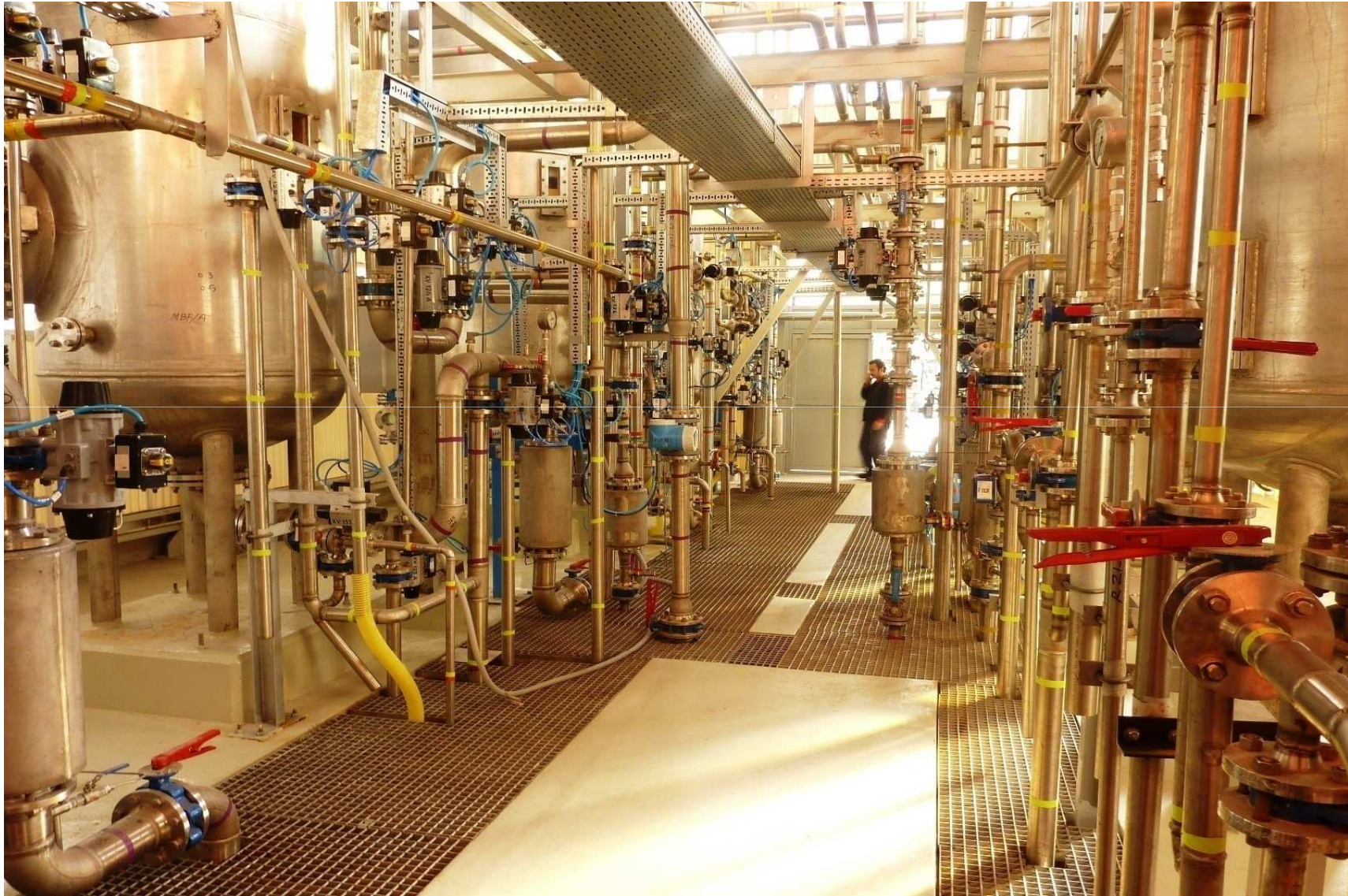
THE FERTAREX ION-EXCHANGE DEMINERALISATION PLANT 60 m 3 /h
